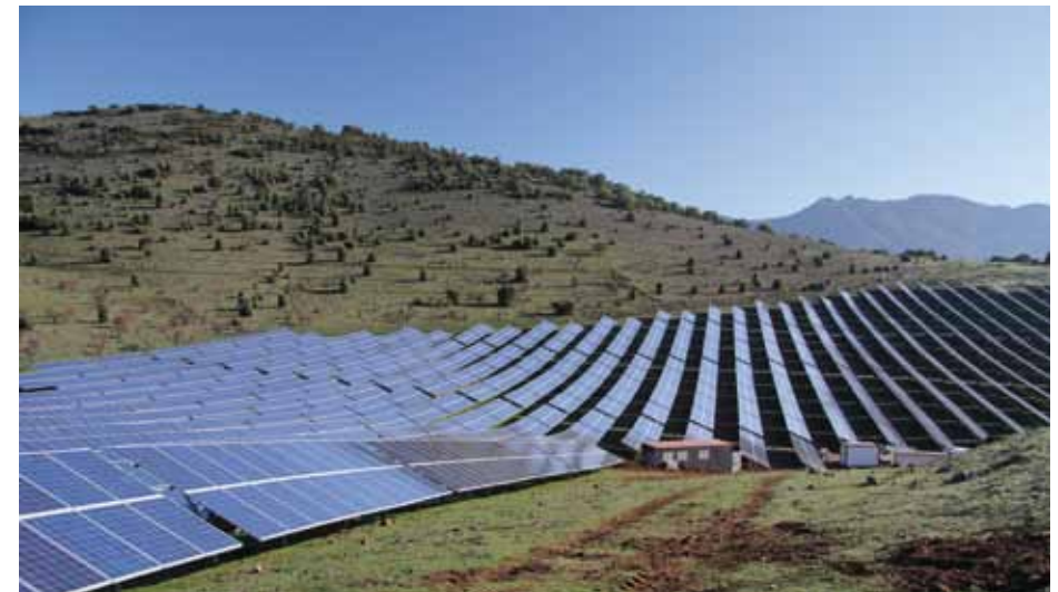
Korsika | France System: 2,6 MW | T-Rack System
